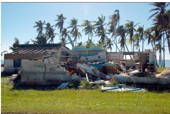
(Above) Te Kaaroa SDA school, Aitutaki after Cyclone Pat struck in early 2010.
